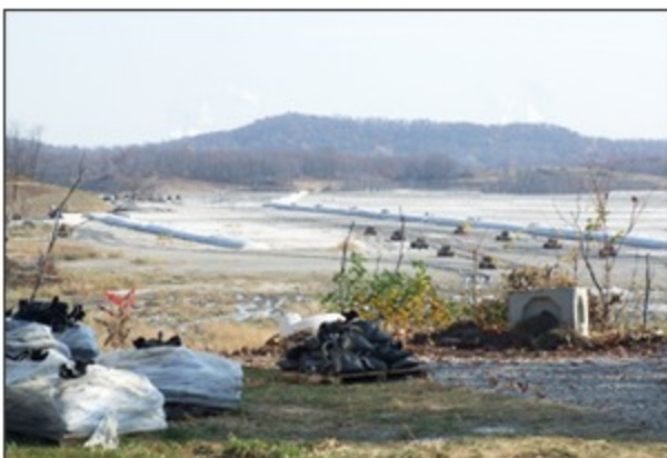
Parts of the Little Blue Run impoundment are visible from nearby neighborhoods.
