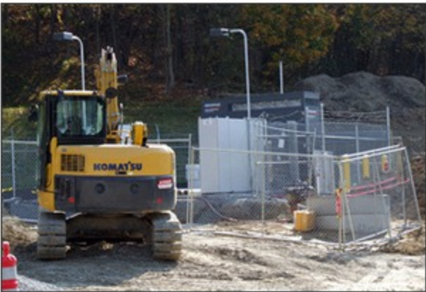
FirstEnergy has installed pumps in Curt and Debbie Havens' neighborhood to control seeps.
